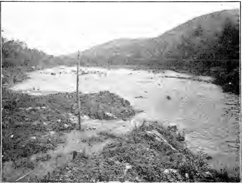
Fig. 2. Carr Pond. Lower extension of lake partly filled, looking northerly from the old dam. (Figures 1 and 2 together cover the greater part of the lake except the section between the old dam and Jacob Riis Camp).
